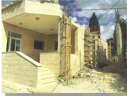
Construction site, in progress
