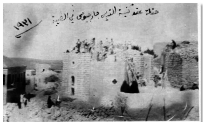
Workers completing the roof
